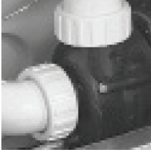
Vent air by slightly opening pump unions.
