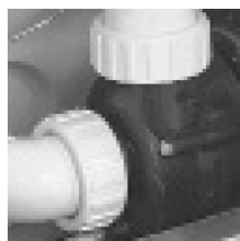
Vent air by slightly opening pump unions.
