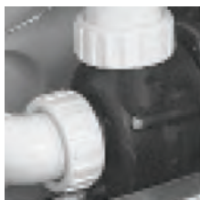
Vent air by slightly opening pump unions.
