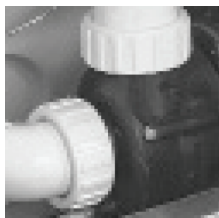
Vent air by slightly opening pump unions.
